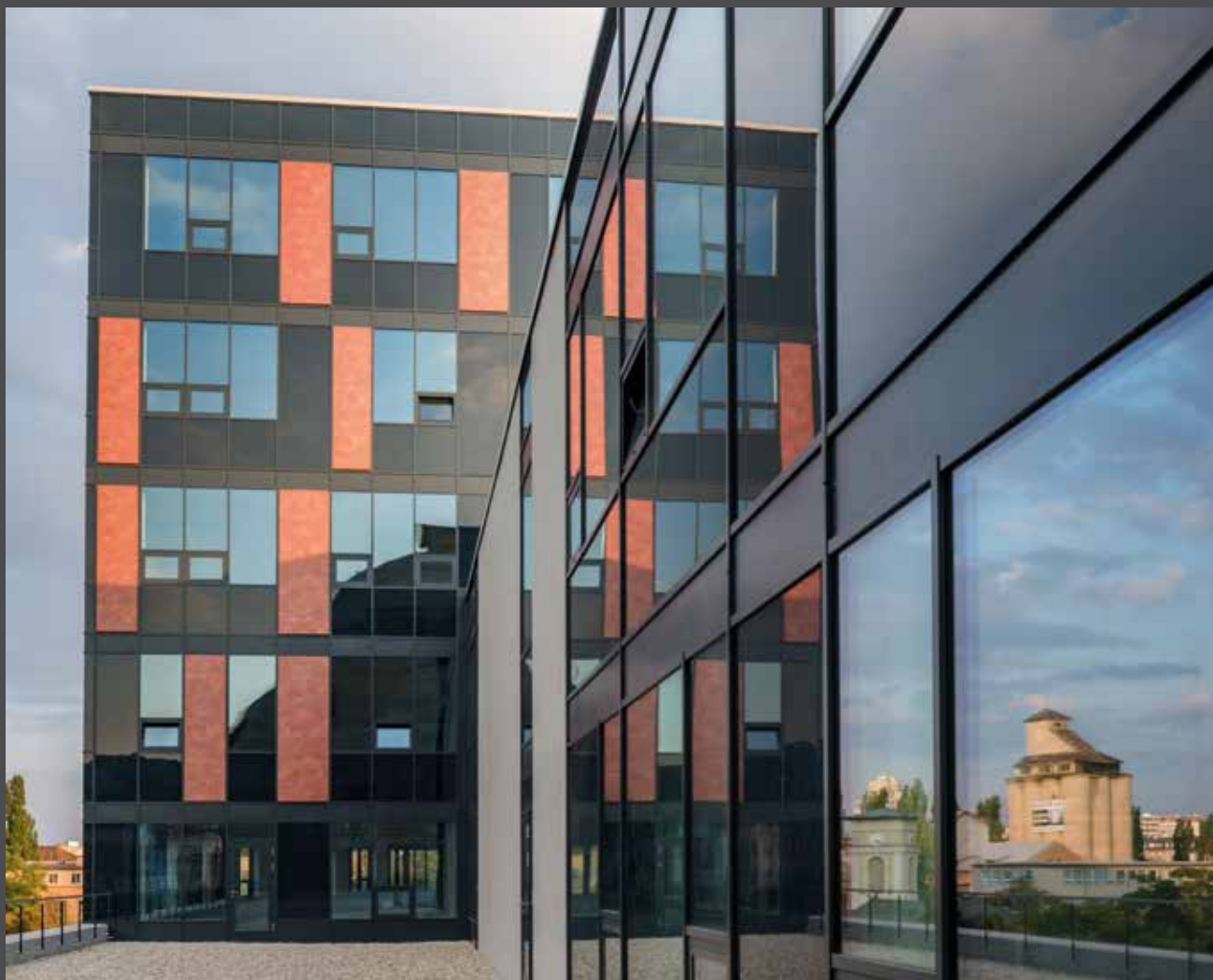
Stein 2 Office Building, Bratislava | Material: ALUCOBOND® PLUS Coracero B mat | Architect: Ateliér Ivan Kubik | Fabricator/Installer: ALUSTEEL © Martin Viazanko
