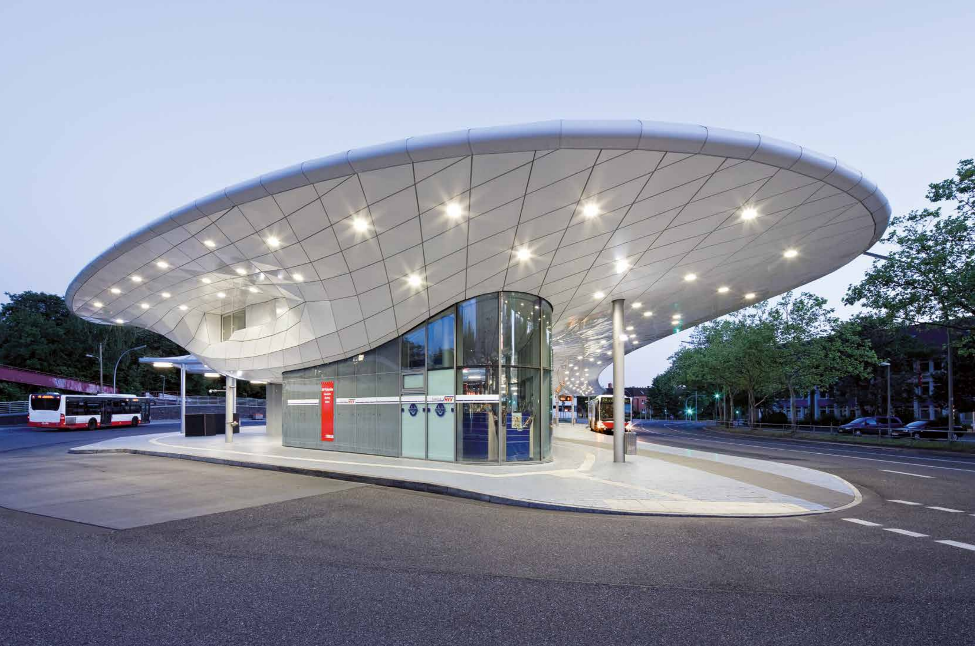
Bus station Hamburg-Poppenbüttel | Blunck + Morgen Architekten, WTM Engineers, Hamburg, Germany
